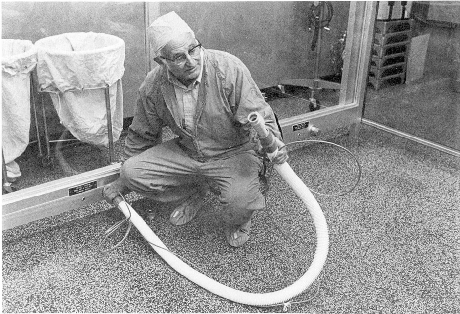
Fig. 2. The vacuum tube is channeled through the lower support of the glass enclosure. Intercom wire is attached to vacuum tube.
