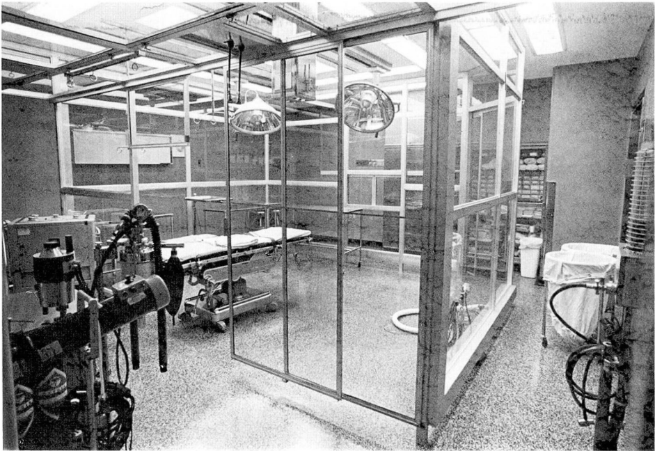
Fig. 1. The glass operating room enclosure at University Hospitals of Cleveland using shatter-proof glass. Vertical air flow about perimeter within the enclosure. Enclosure elevated 4 inches from floor to provide air outlet. Sliding doors provide entrance room for patient and surgical team. Sliding glass instrument pass window for circulating nurse.
